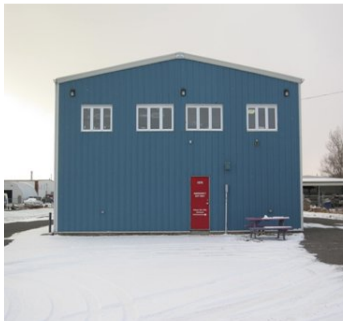
Minor Fisheries processing facility
